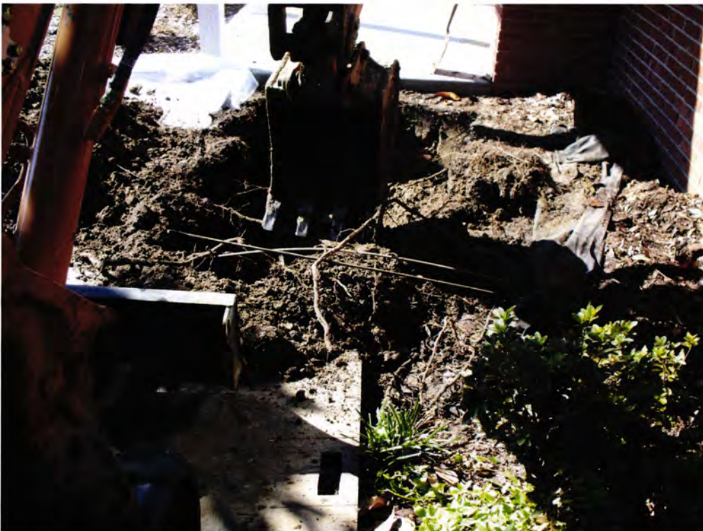
Picture 2: UST 475Dogwood-1 excavation in progress.
